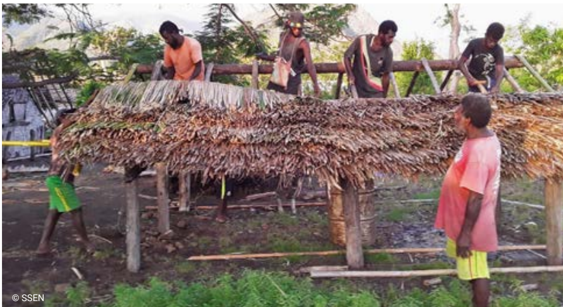
Community members construct a hurricane house.
